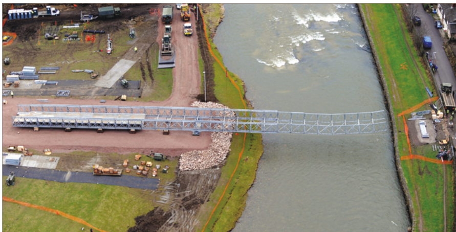
Figure 7. Aerial view showing the 92 t structure being winched across the river – the upward curve of the lightweight nose sections compensates for the 1.4 m deflection
