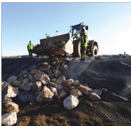
Figure 5. Limestone riprap was used to protect the southern abutment from 1-in-100-year floods
