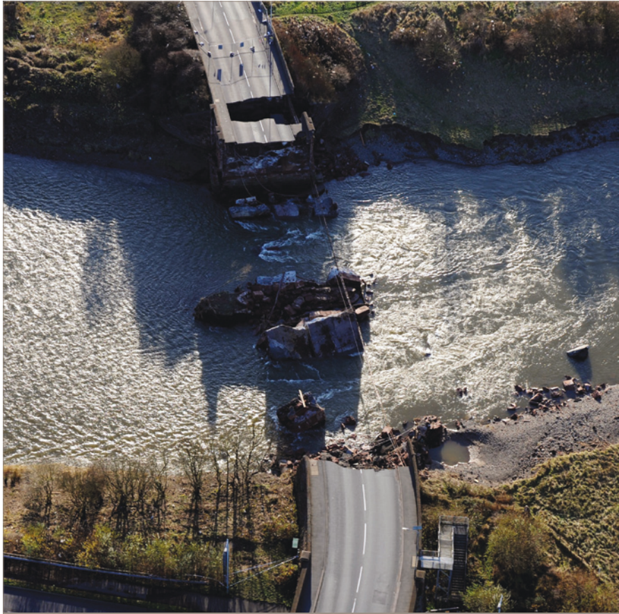
Figure 2. The A597 Northside Bridge over the River Derwent in Workington collapsed on the afternoon of 20 November 2009, killing police officer Bill Barker
