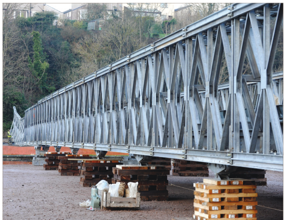
Figure 4. The logistic support bridge is made from standard steel truss panels and then launched from rollers on a geotextile-reinforced construction platform
